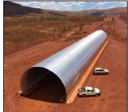
Trinity Drive Overpass, Solomon Mine, FMG, WA
