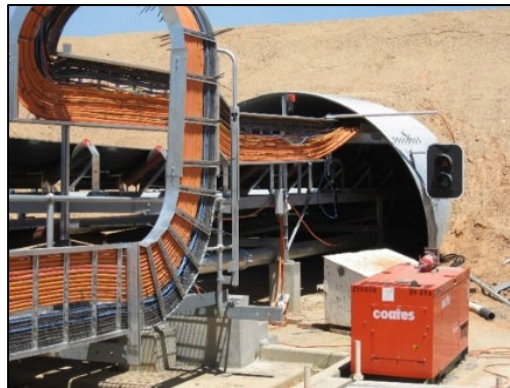
Lake Vermont stockpile conveyor tunnel – B200
