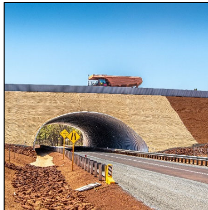
Large-span arch – Lower Hotham Rd, South32, WA.
