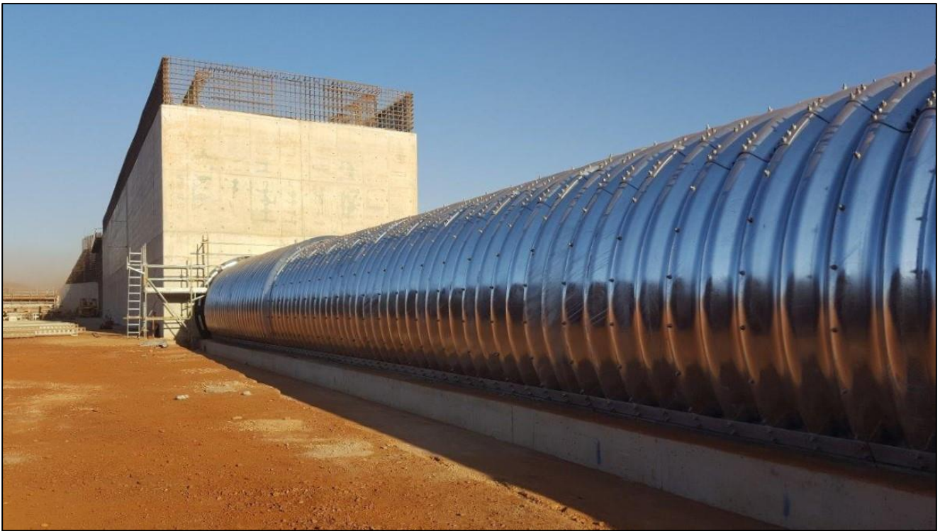
BHP Mining Area C stockpile tunnel
