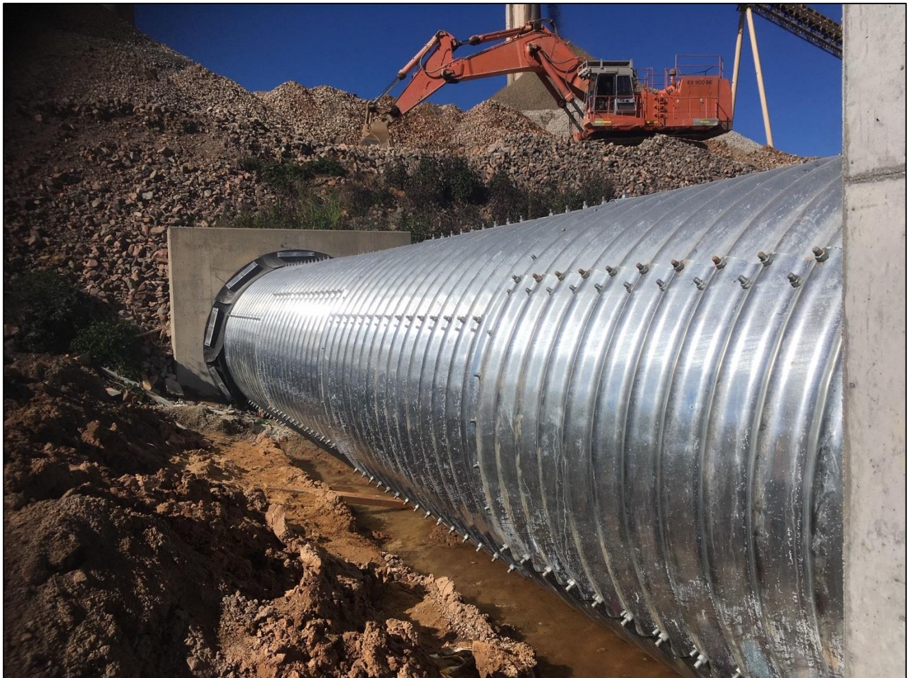
North Parkes Escape tunnel extension
