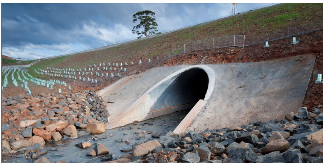
Dilston Bypass, Launceston, Tasmania
