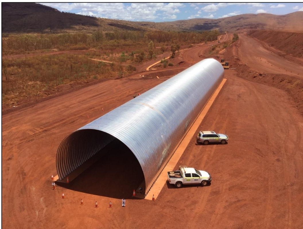
FMG's Trinity Drive Overpass – assembled in 2 weeks.
