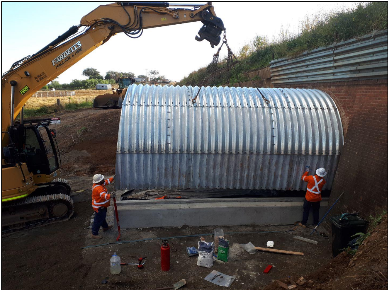
Nemingha Culvert extension
