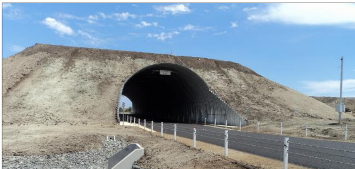
Large – span arch at Baralaba Road, Anglo American Coal, Dawson Mine site, QLD – during construction and during backfilling
