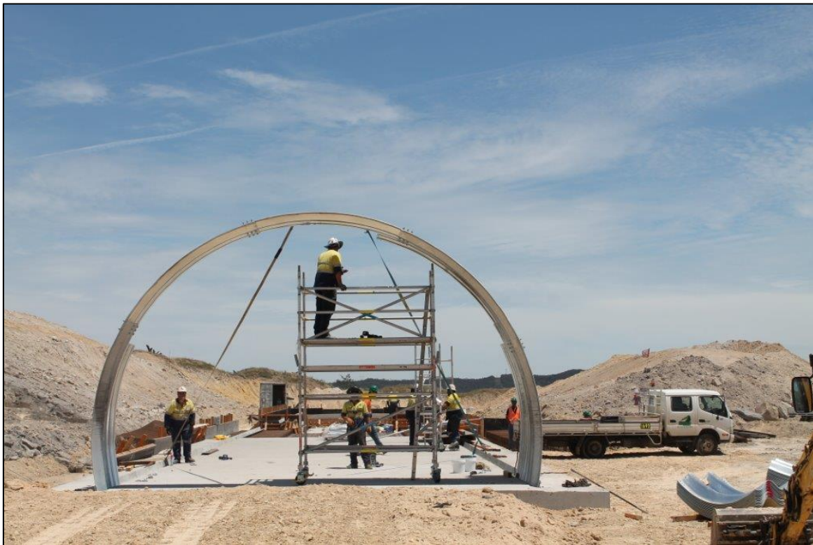
Moolarben Coal – Conveyor Tunnel / Haul Road Underpass 2015
