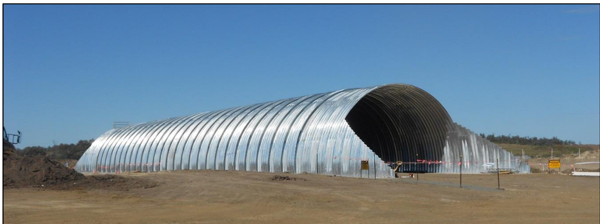
Large – span arch at Baralaba Road, Anglo American Coal, Dawson Mine site, QLD – during construction and during backfilling
