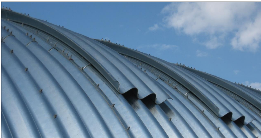
Detail of external ribs – Gibihi Road, Qld
