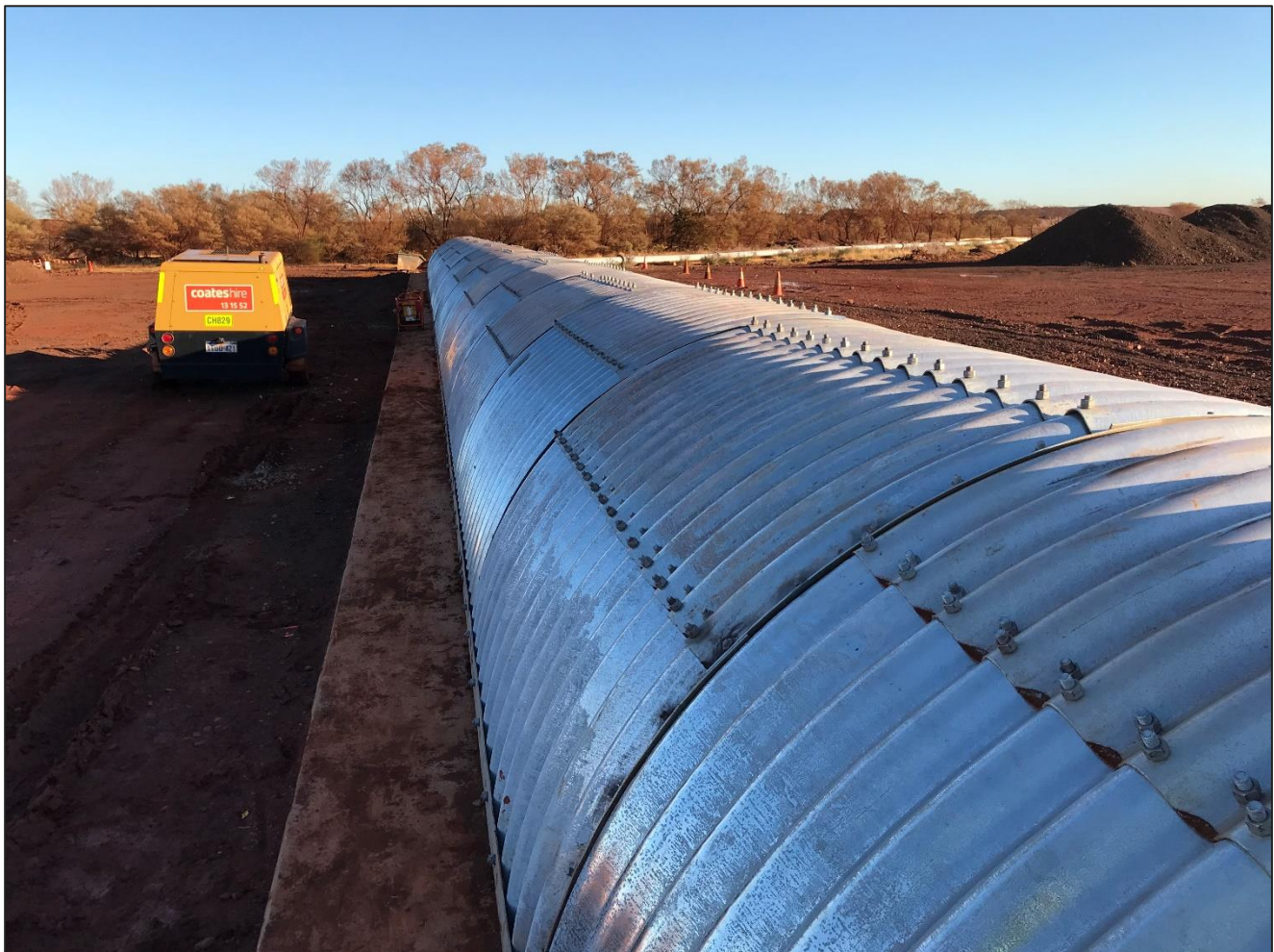
FMG Tailings Dam B200
