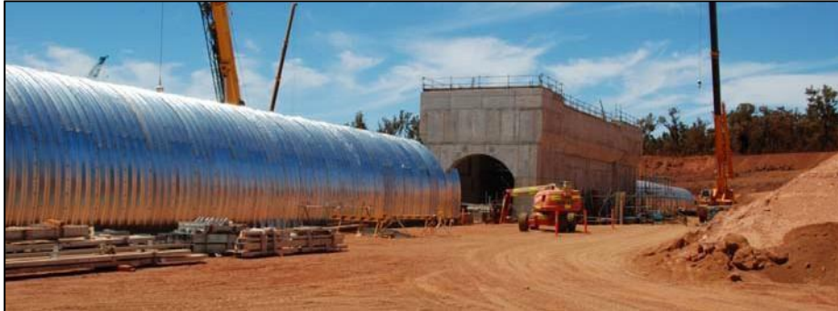
410E Stockpile Tunnels – BHP Worsley Efficiency & Growth project, Marradong, WA.
