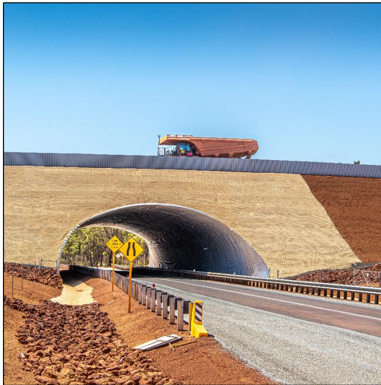
Large-span arch – Lower Hotham Rd, South32, WA.
