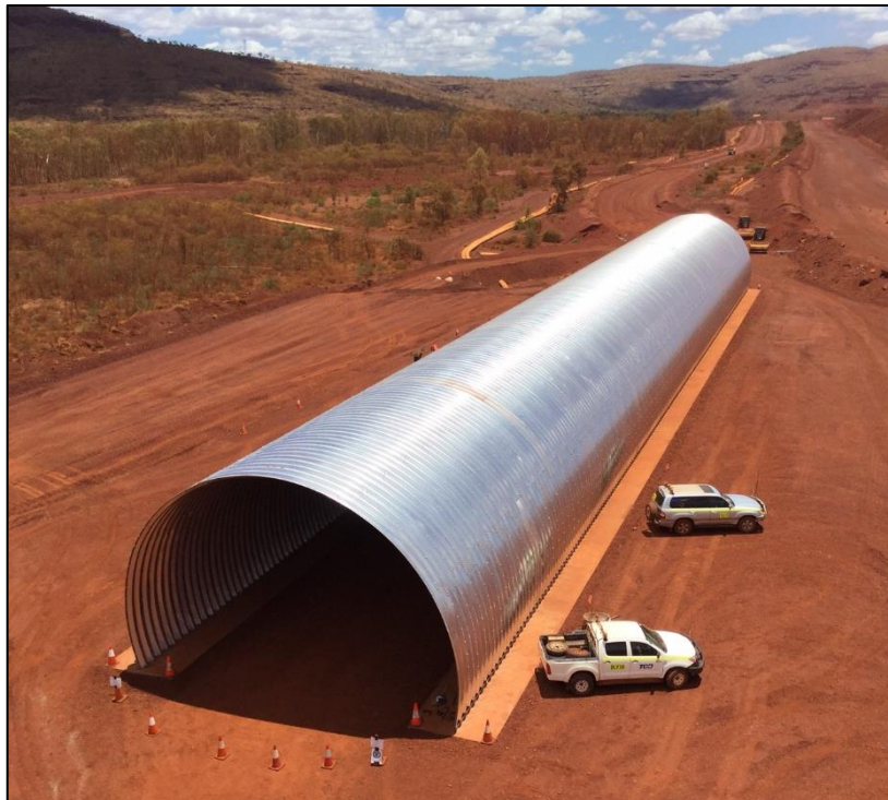
Trinity Drive Overpass, Solomon Mine, FMG, WA
