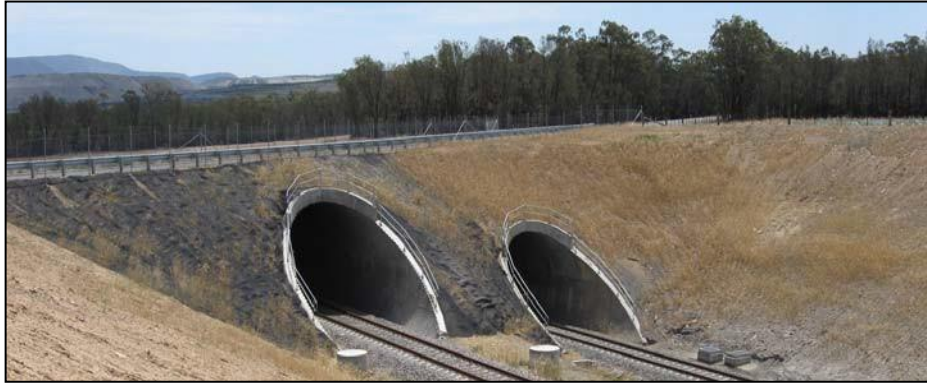
B200 multi-plate structures, Wambo Rail Spur, NSW
