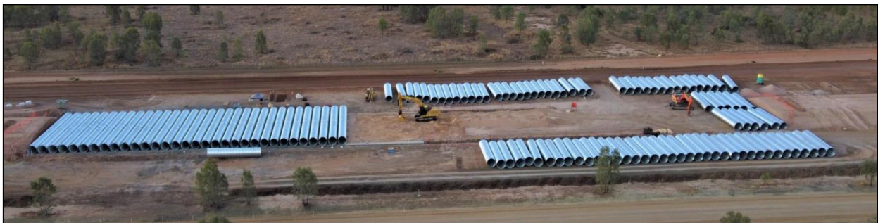
Carmichael Rail project, Bravus (Adani), QLD
